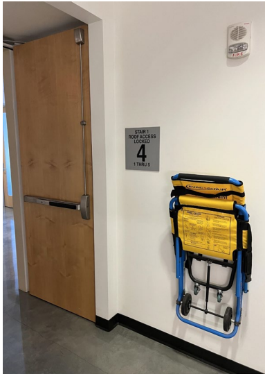
Figure 1: In Stairway 4 (4-1) (E)
